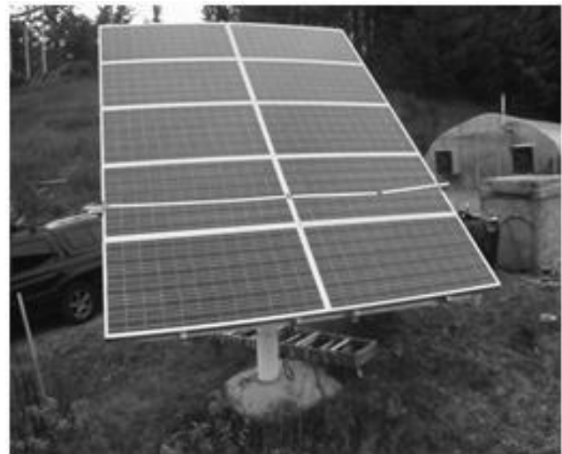
Fig. 1: A photo of the two arrays showing the shading.
